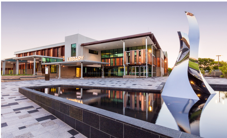
Library forecourt with seamless connection to civic square. Plaza areas designed to accommodate civic/community events. Bespoke art piece in foreground "Confluence".
