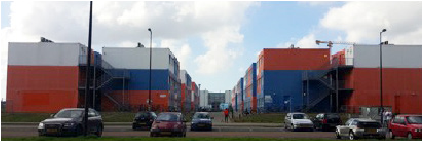
High-density modular living made with shipping containers. Note the vibrant colours creating a contemporary feel. Amsterdam North, 2016.
