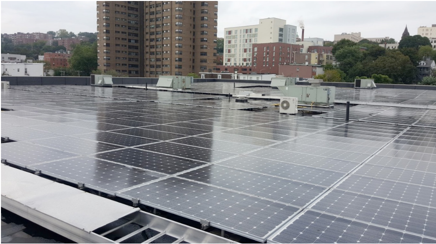
Solar panel array on top of a roof of a municipal building.
