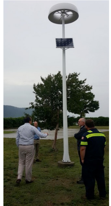
Mr Luis Barros from Omniflow explains the operation of Omniled smart lighting tower.
