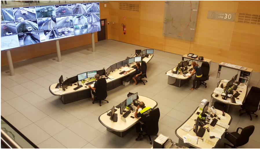
M30 Calle control centre – a very modern facility.
